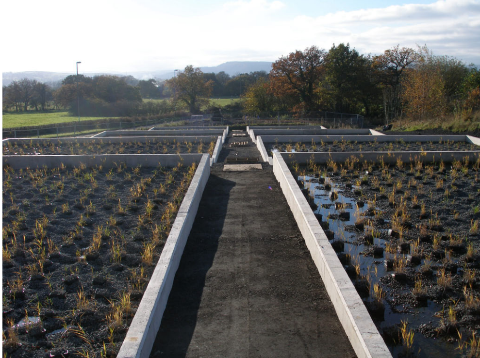
Construction of Reed Beds
