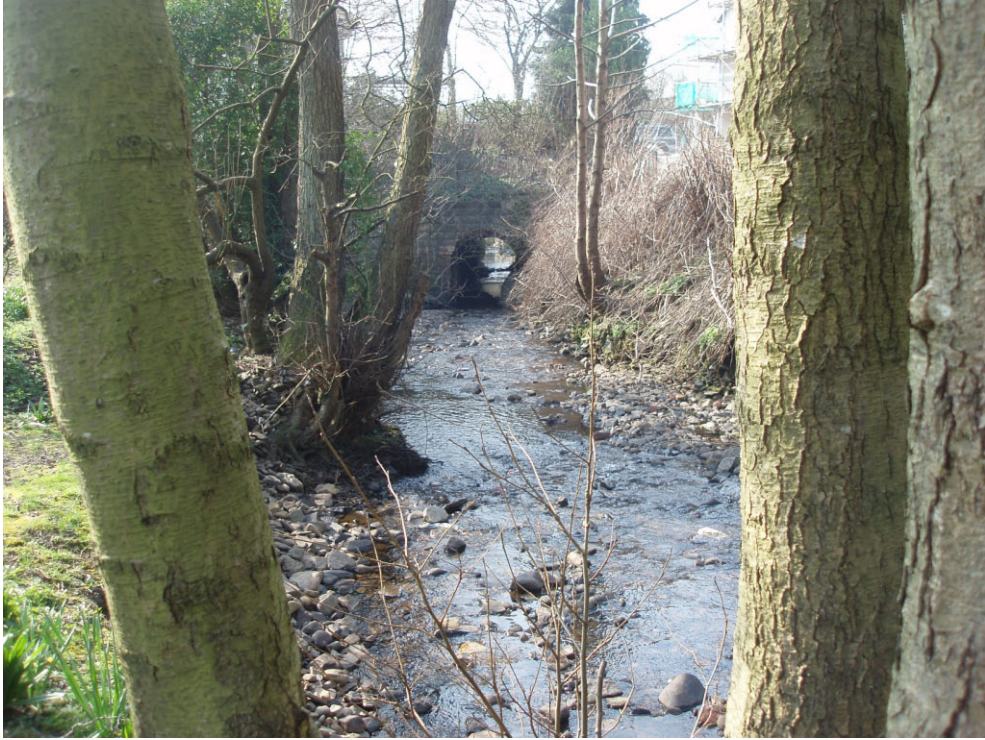
Natural Watercourse and Culvert
