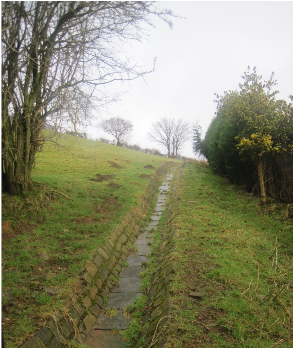
Matured Drainage Channel
