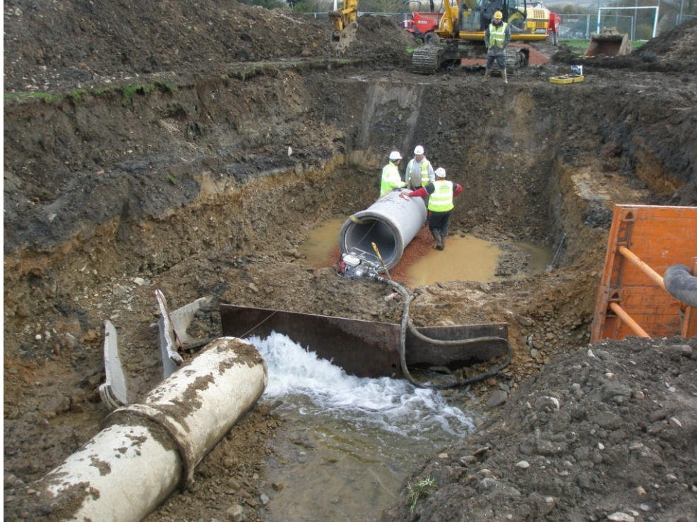
Sub-standard culvert being replaced
